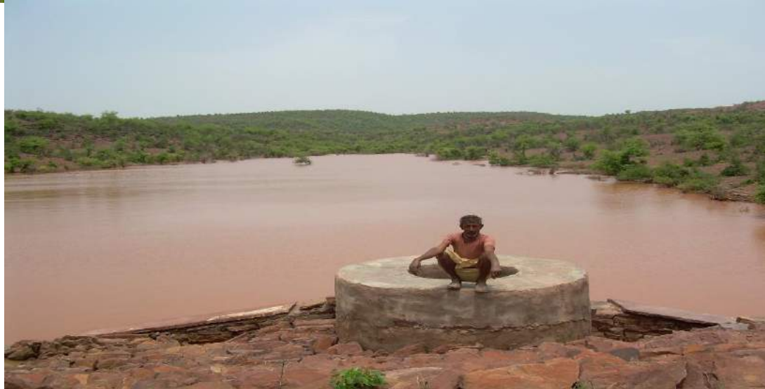
Pictures of various types of structure constructed by GGS
