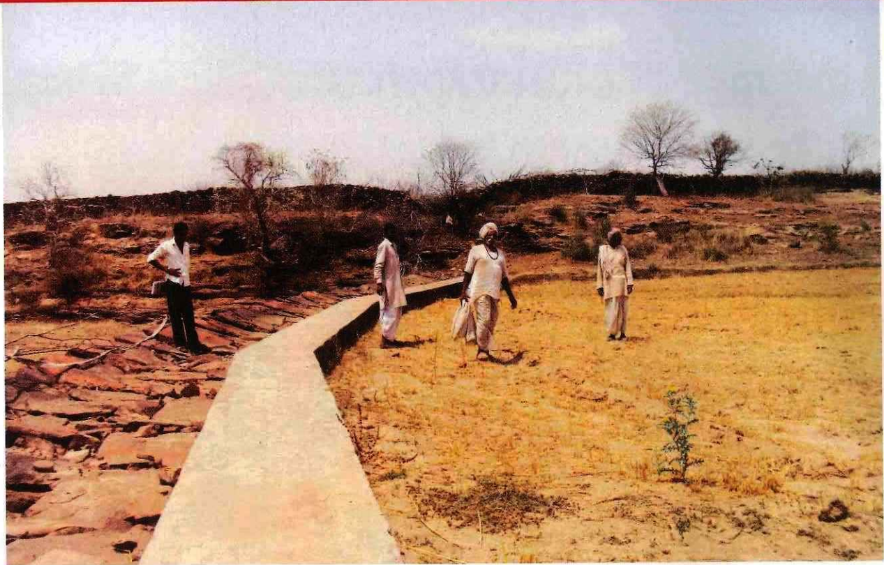
(Above) Concrete pagaraa, a soil conservation structure, built next to kuchcha pagaraa in Nivera village; Rock paintings in Albati village show pagarra-like structures
